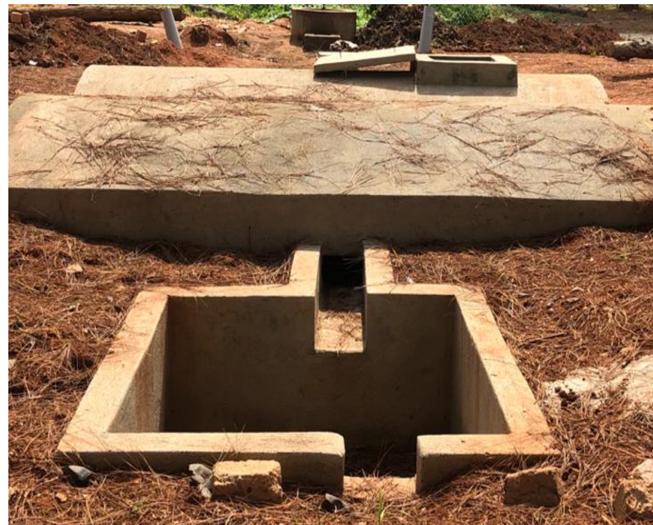
BIODIGESTER CONNECTION
