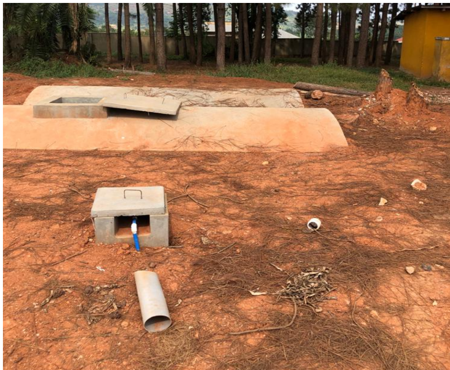
BIODIGESTER CONNECTION
